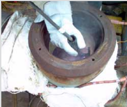
Thermal power plant - control valve seat replacement
