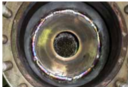
Surfacing of the valve seat
