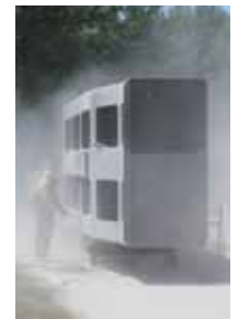
Sandblasting of hydropower dam shutter
